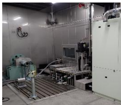
Engine Test Equipment
