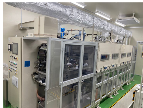
Coating equipment installed in a dry environment
